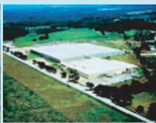
McQuay Auburn Factory, USA
