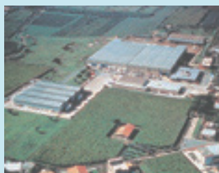
European Manufacturing Base of McQuay Air-cooled Heat Pump in Cecchina Italy
