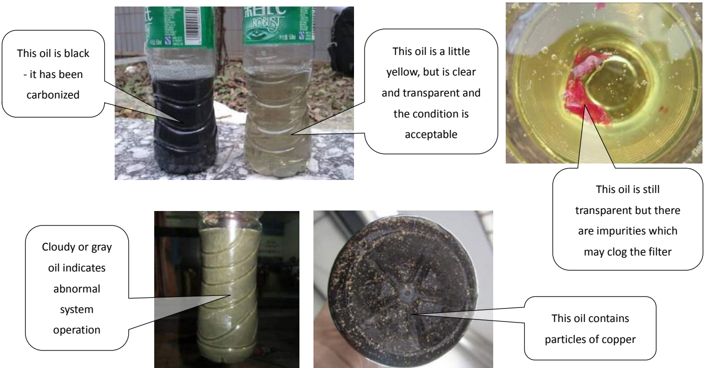
Figure 5-4.16: Inspecting compressor oil
